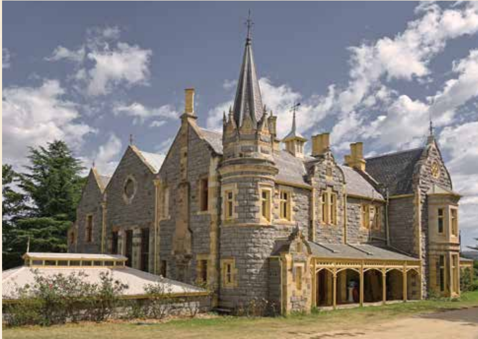
Of note are the restored chimney stacks, the tower with gables and 'candle-snuffer' roof, and the Hawkesbury sandstone trim contrasting with the grey granite and black tuck pointing. The low building at left was originally a glass-roofed greenhouse, destroyed in a hailstorm in the 1880s. The roof was rebuilt in 1980s. Future plans include reconstruction of the glass roof. Photo, GL
