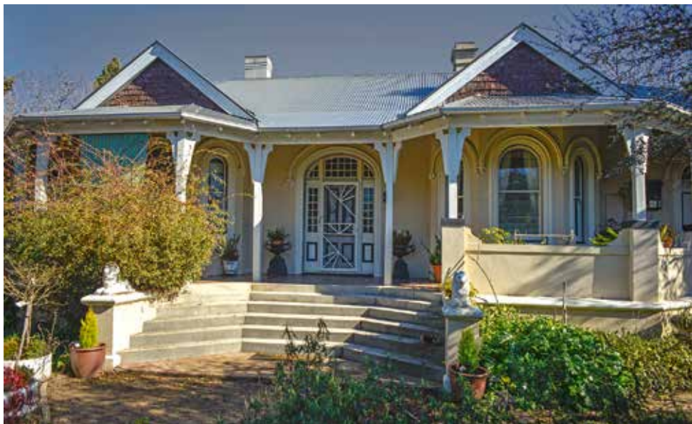
The home, Glendower , built by Jones in 1882–84 for Lewis Lloyd MLA, on Lloyd's Road, South Bathurst. After a fire swept through the top floor in 1913, the house was rebuilt by John Copeman. The Federation-style verandah now contrasts with the original Victorian stucco trim and Gothic bosses. Photo, GL
