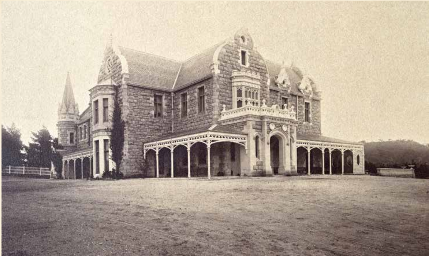
The Mount , from the north-east, c1885. 'Lizzie's corner', under the verandah, is where James Rogers buried the time capsule. Note the balustrade over the porch is of a lighter coloured and less durable sandstone, possibly local soapstone. Photo, Kerry and Jones, Photographers, Sydney, BDHS
